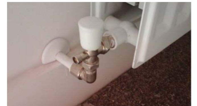
Standard valve with drain point
